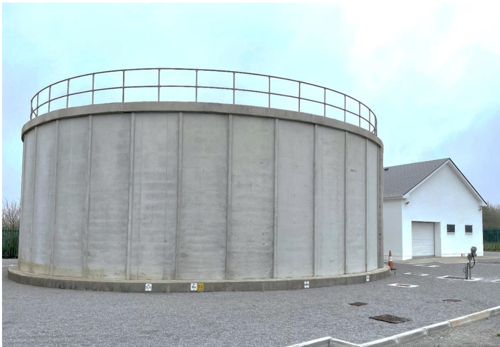
Tuam RWSS Extension to Loughrea - Completed reservoir and pumping station at Seefin
