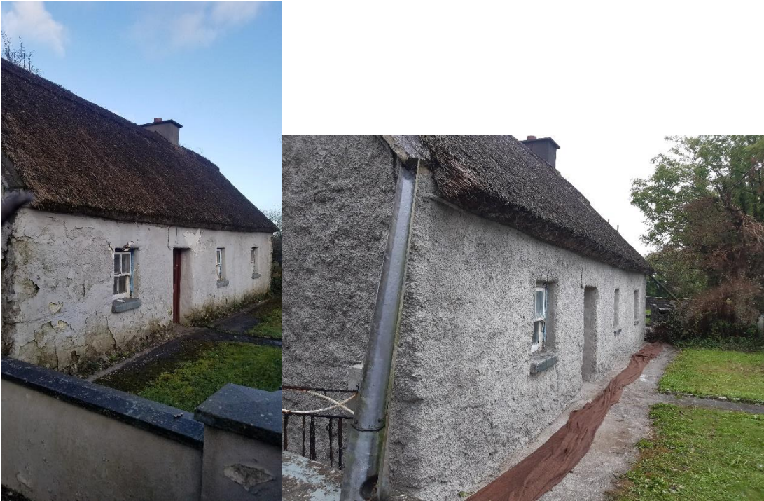
Repair to lime render, Cluidrevagh
