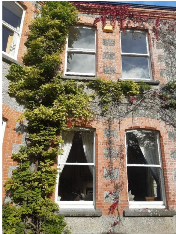
19 th Century timber sash windows repaired at Lissbeg House.
