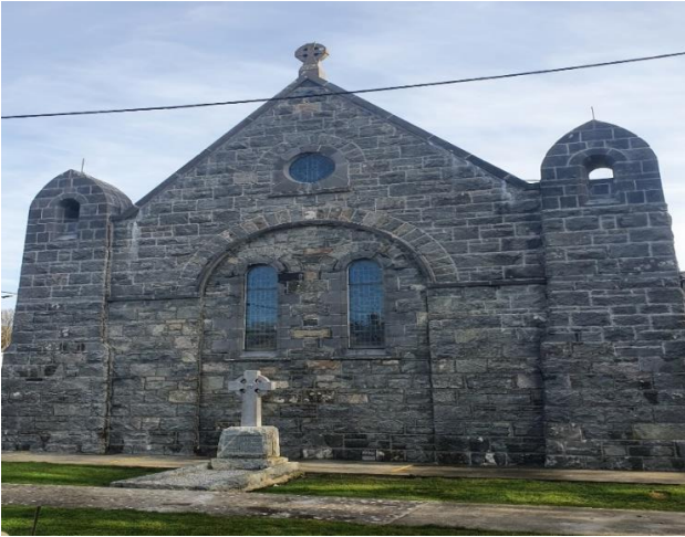
Cill Einde An Spideal, repairs to masonry and roof
