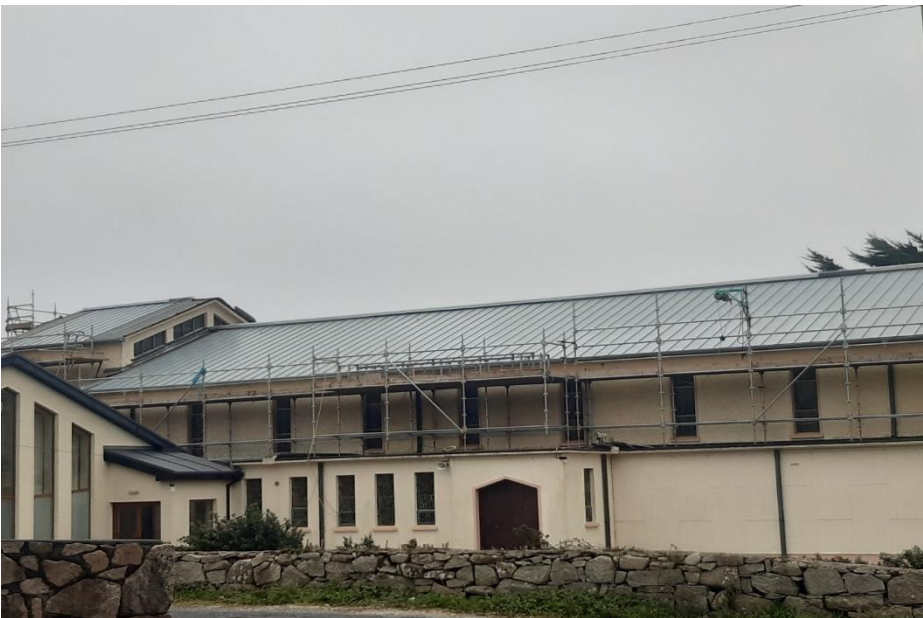
Leitirmoir ; Repairs to roof to prevent water ingress
