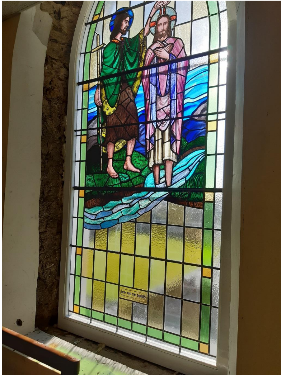
Stained glass window repair St Patrick's Church, Derrybrien.
