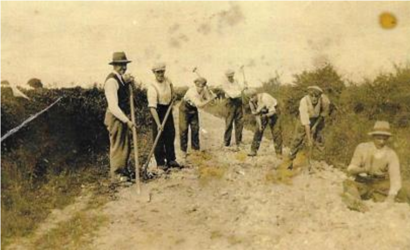
Sepia photograph depicting 6 roads workers with picks, sledgehammers and shovels, and a Ganger (Supervisor) on the left-hand side, c. 1925 [Ballygar district], GS21/01.
