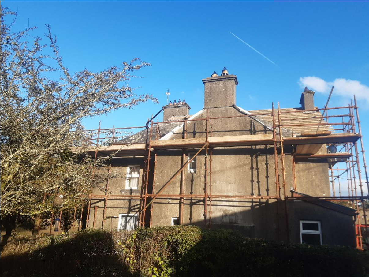
Repairs to roof of The Bay, Woodford
